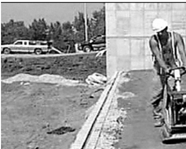
Backfill and compact
