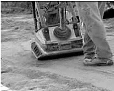
Backfill and compact
