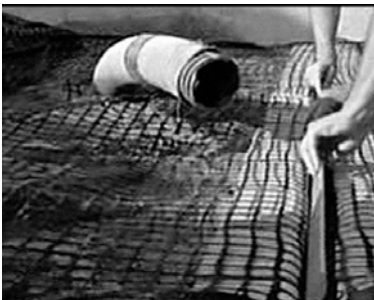
Lock bar installation
